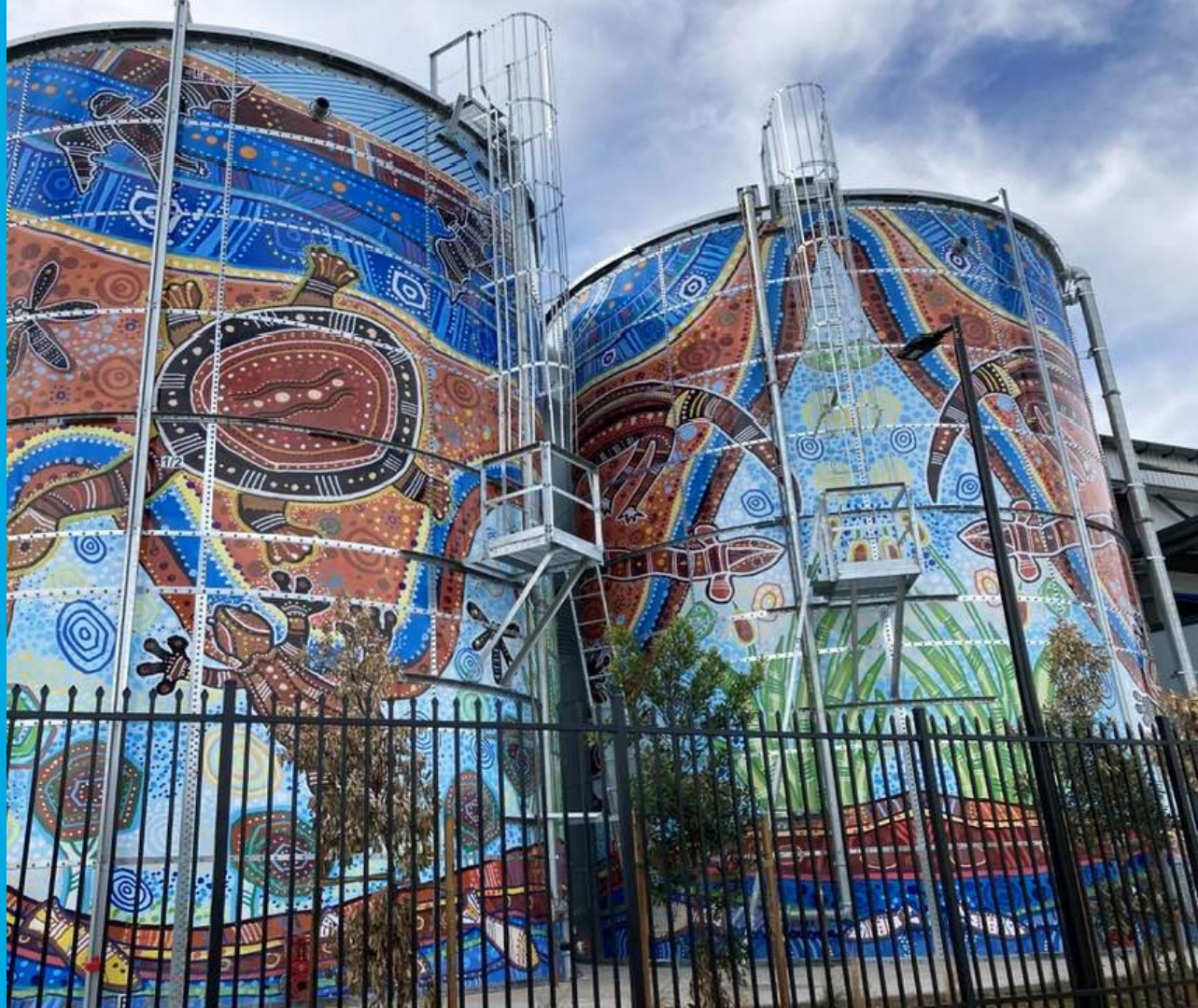
Pictured: Western Sydney MRF water tanks
