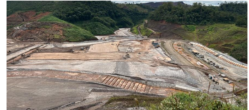
Germano dam decommissioning process
