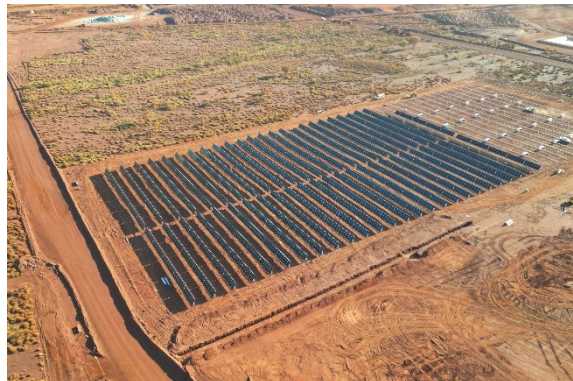
Solar array under construction at Ken's Bore
