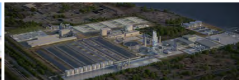
Investing in low-carbon technology Supplying high-grade direct reduction iron ore pellets to GravitHy from 2028
