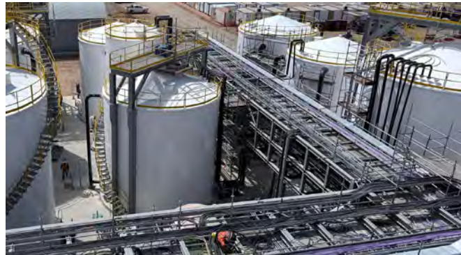
Progress by October 2024
