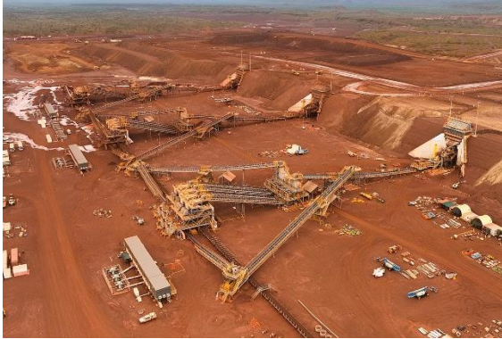
All three MinRes NextGen crushers at Ken's Bore
