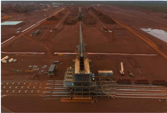
Truck loadout (TLO) facility
