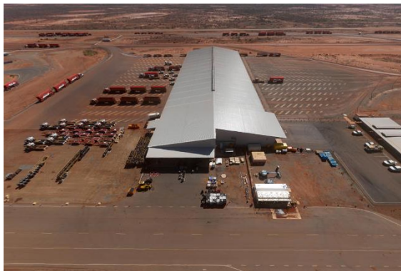
Truck maintenance facility
