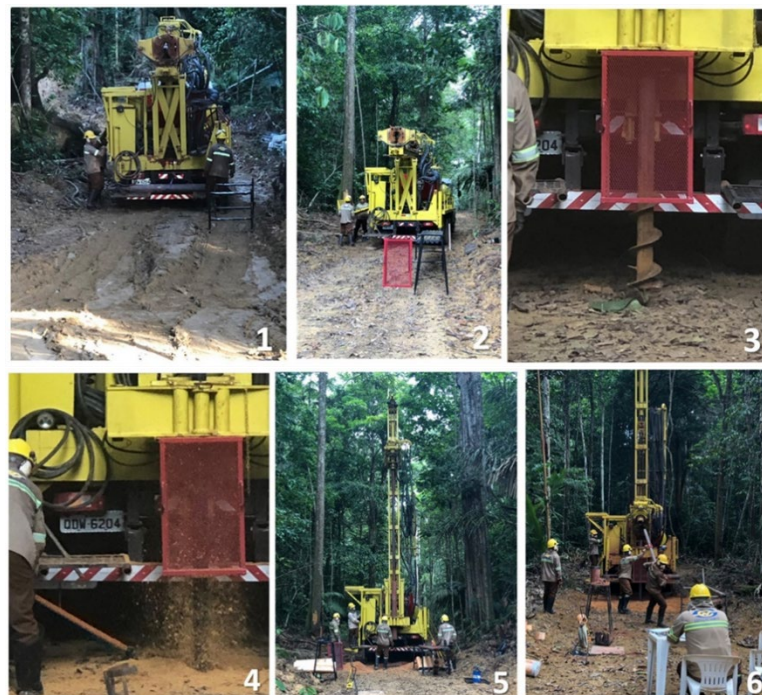
Figure 24 Drilling operation in MRN plateau
