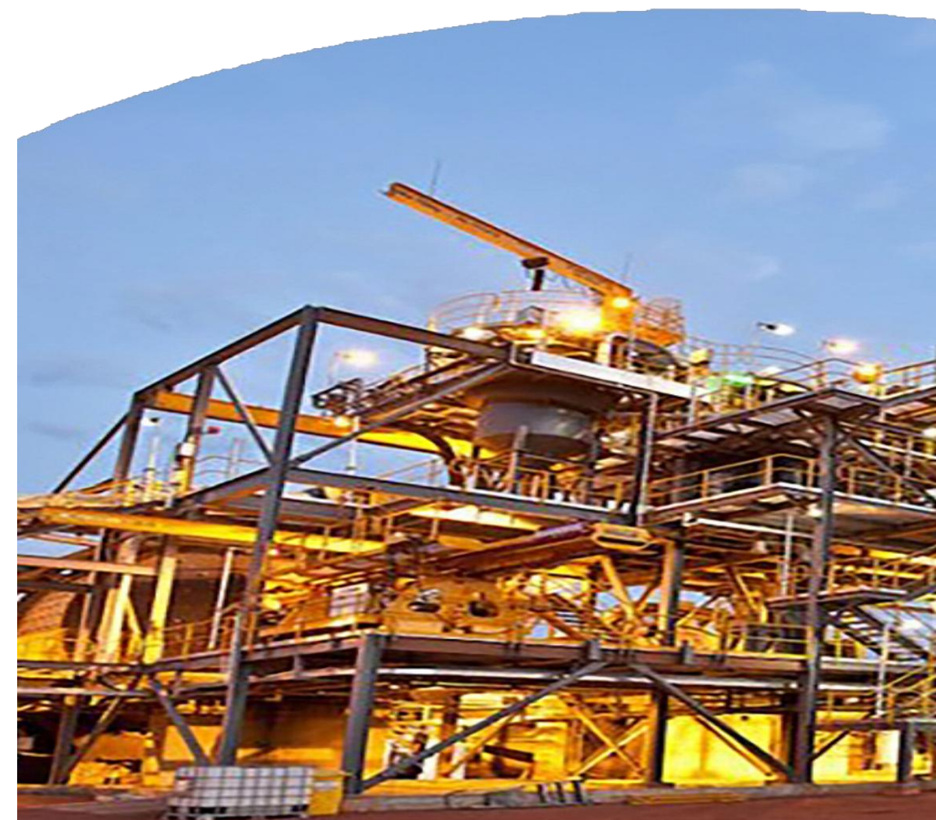
DeGrussa Processing Plant
