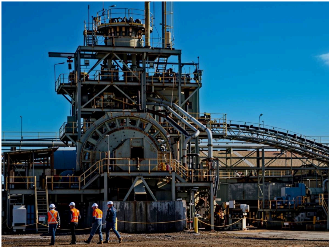
Figure 2: Edna May Processing Facility
