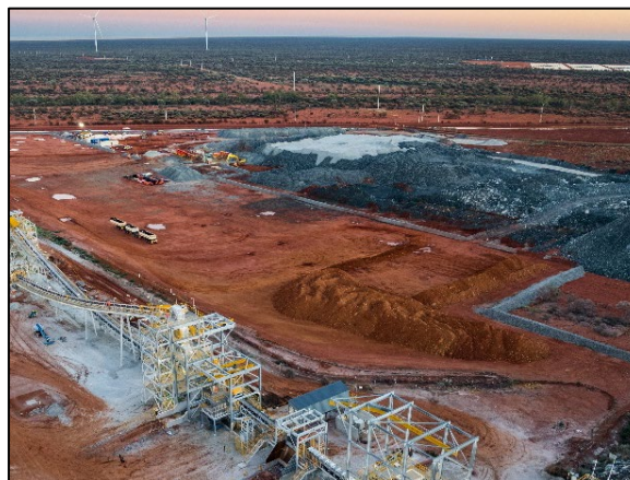
Figure 8: Waste rock crushing and earthworks for permanent Mine Services Area
