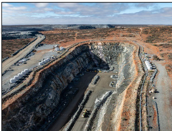
Figure 7: Infrastructure preparation at North-West Flats
