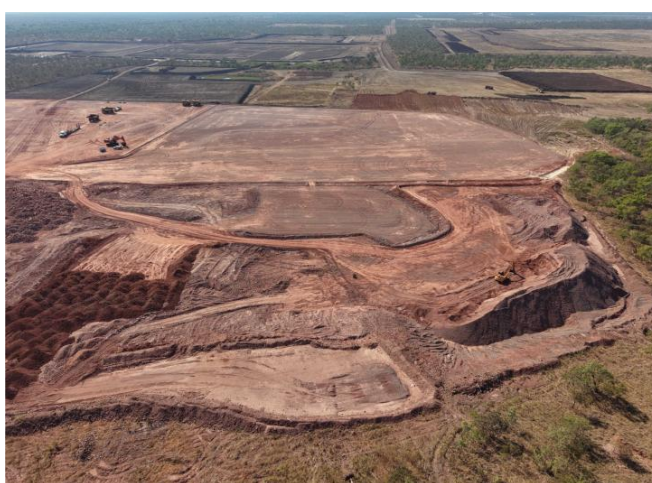
Figure 4: On site quarry with the process plant pad behind it.
