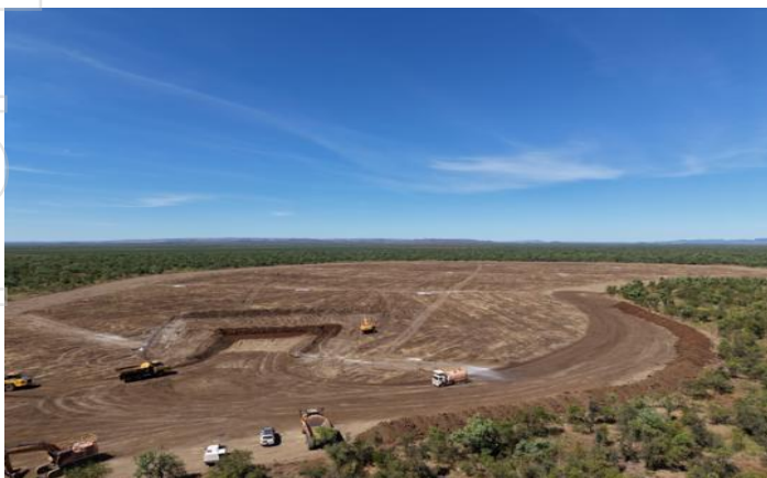
Figure 5: Excavation of B Pit
