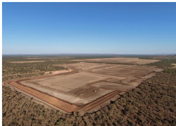
Figure 6: Evaporation Pond Construction
