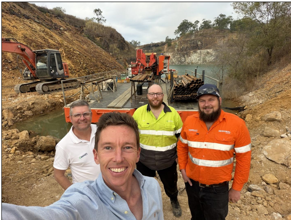
Figure 3 – Diamond rig successfully craned onto the pontoon ready to commence drilling.
