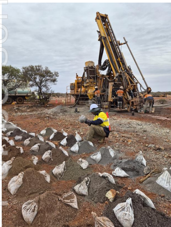
Figure 2: Drill rig operating on site at Ricci Lee
