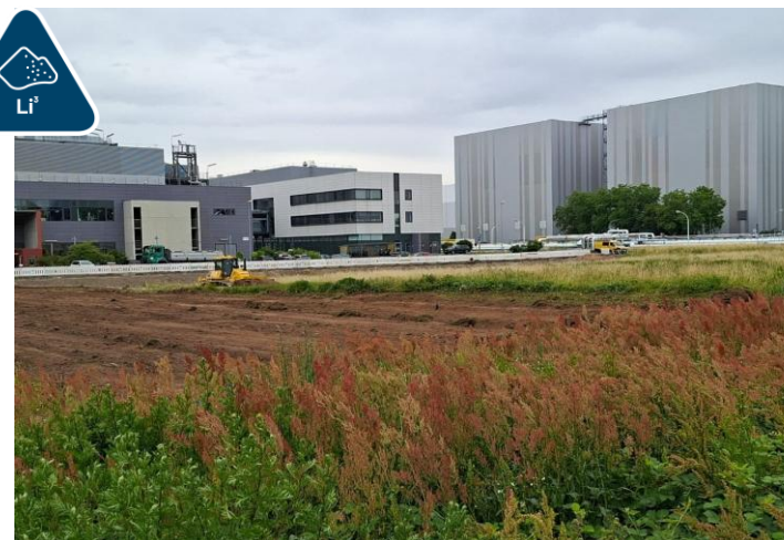
Early bulk earthworks at the Frankfurt lithium chemical plant site
