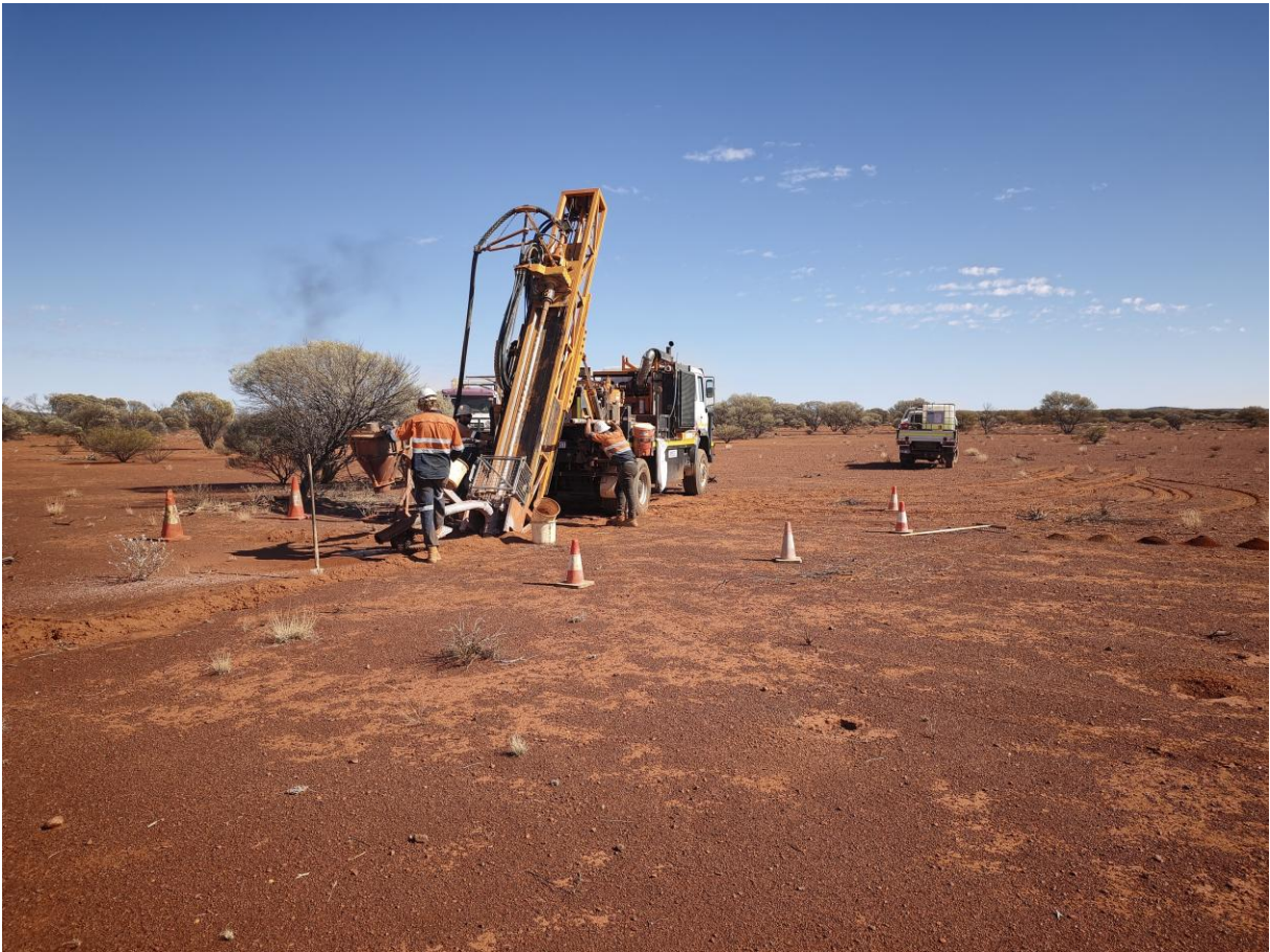
Figure 1 : Air Core drill rig on site at Morck Well
