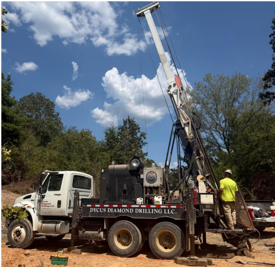
Figure 2. Dycus Rig on site at the first hole.
