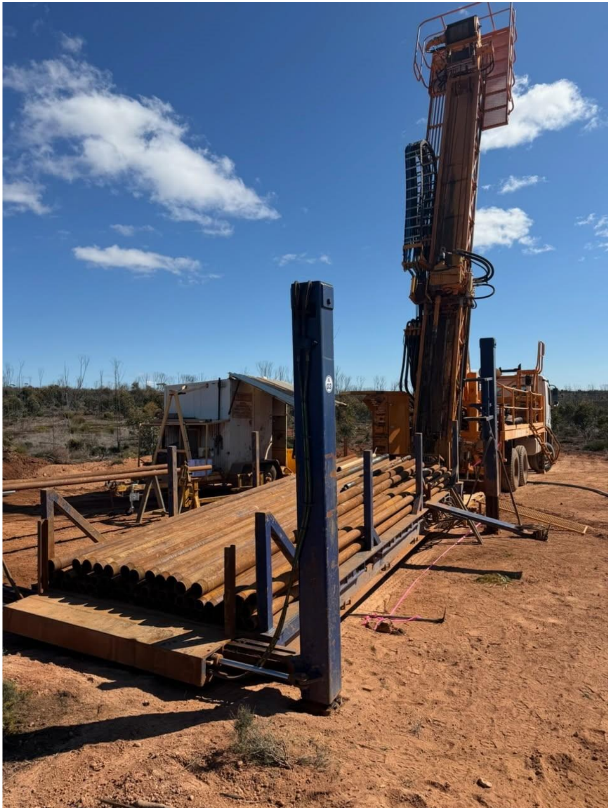
Figure 1 – Drilling Rig setup on first drillhole
