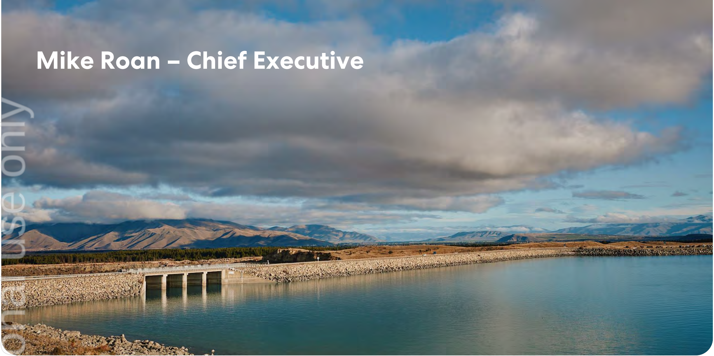
Control structure and spillway, Lake Pūkaki
