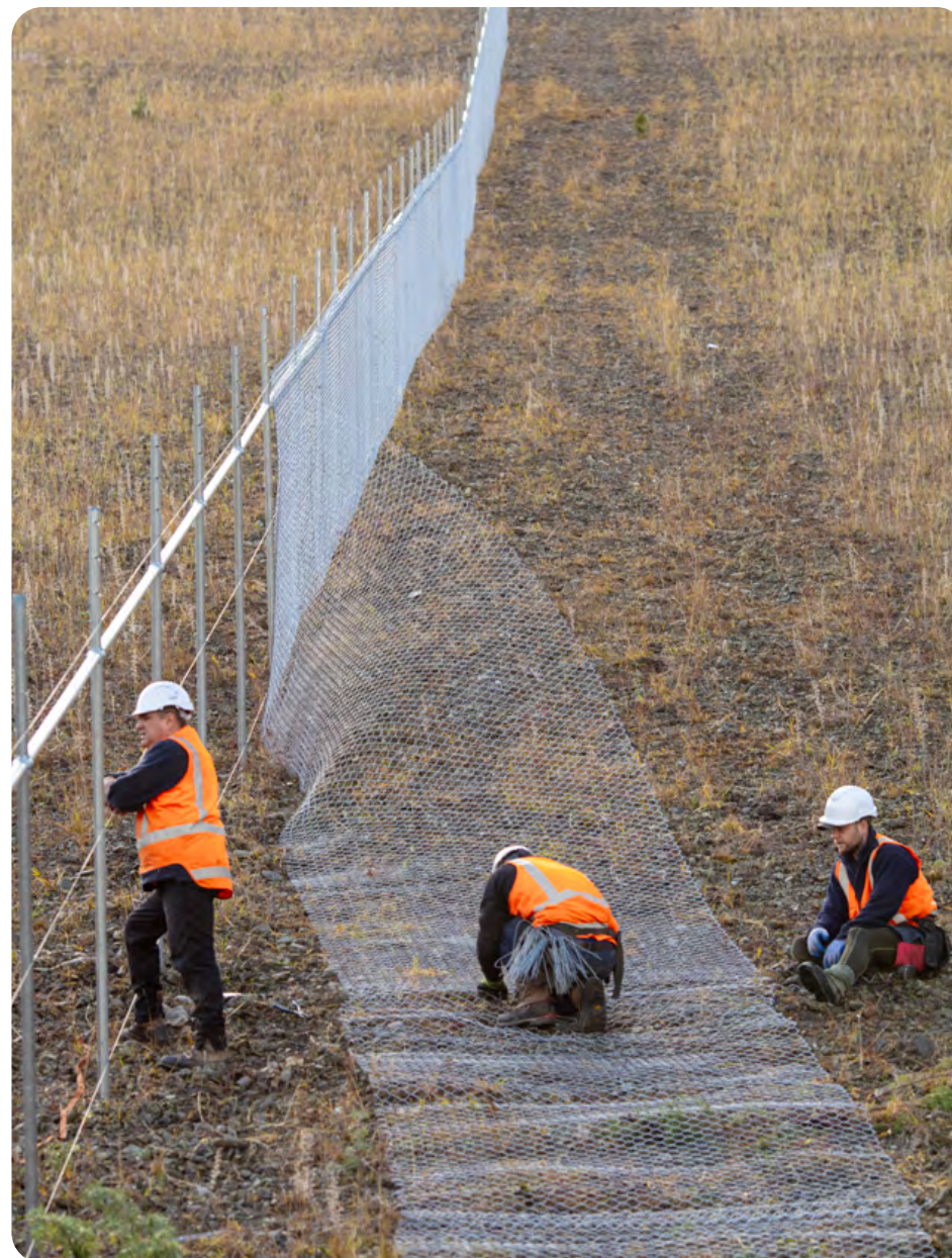
ABOVE: Fencing installation Benmore Power Station, Ōtematata.
