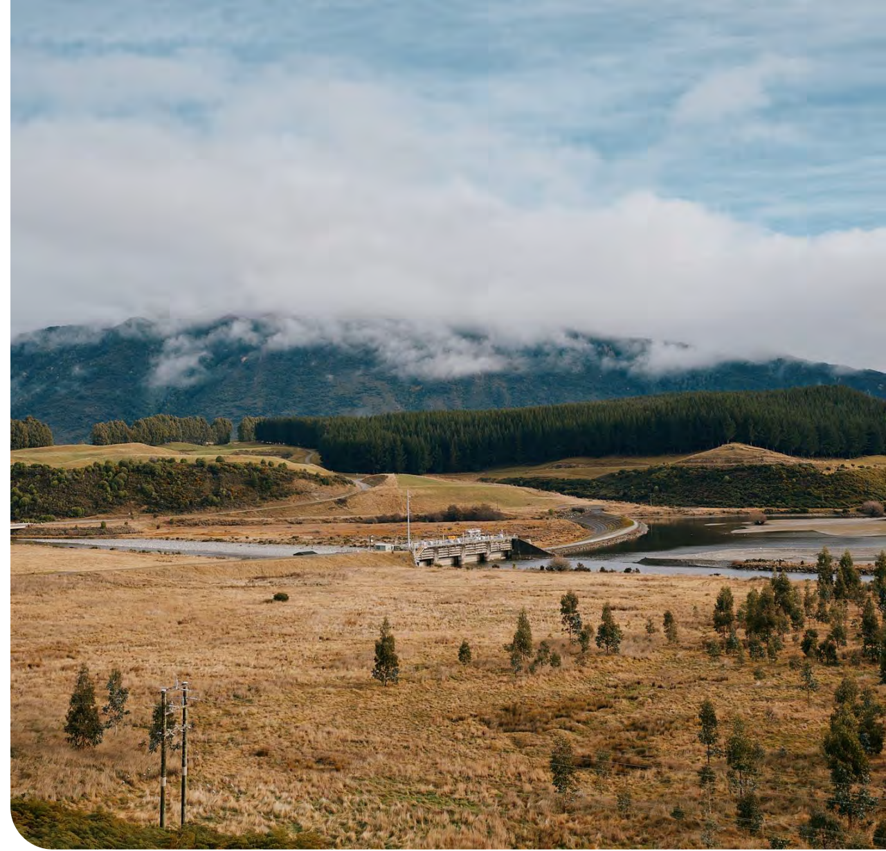
Manapōuri Lake Control structure
