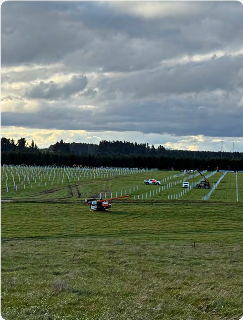
ABOVE: Te Rahui Solar Farm under construction.
