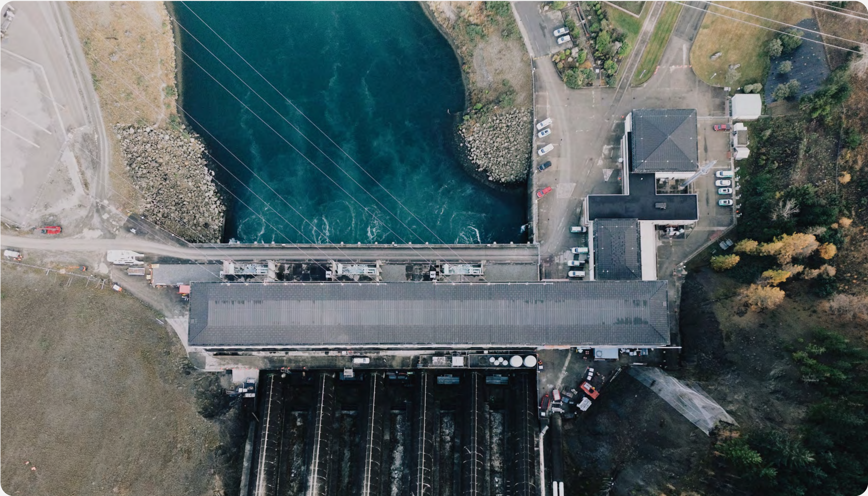
ABOVE: Benmore Power Station.
