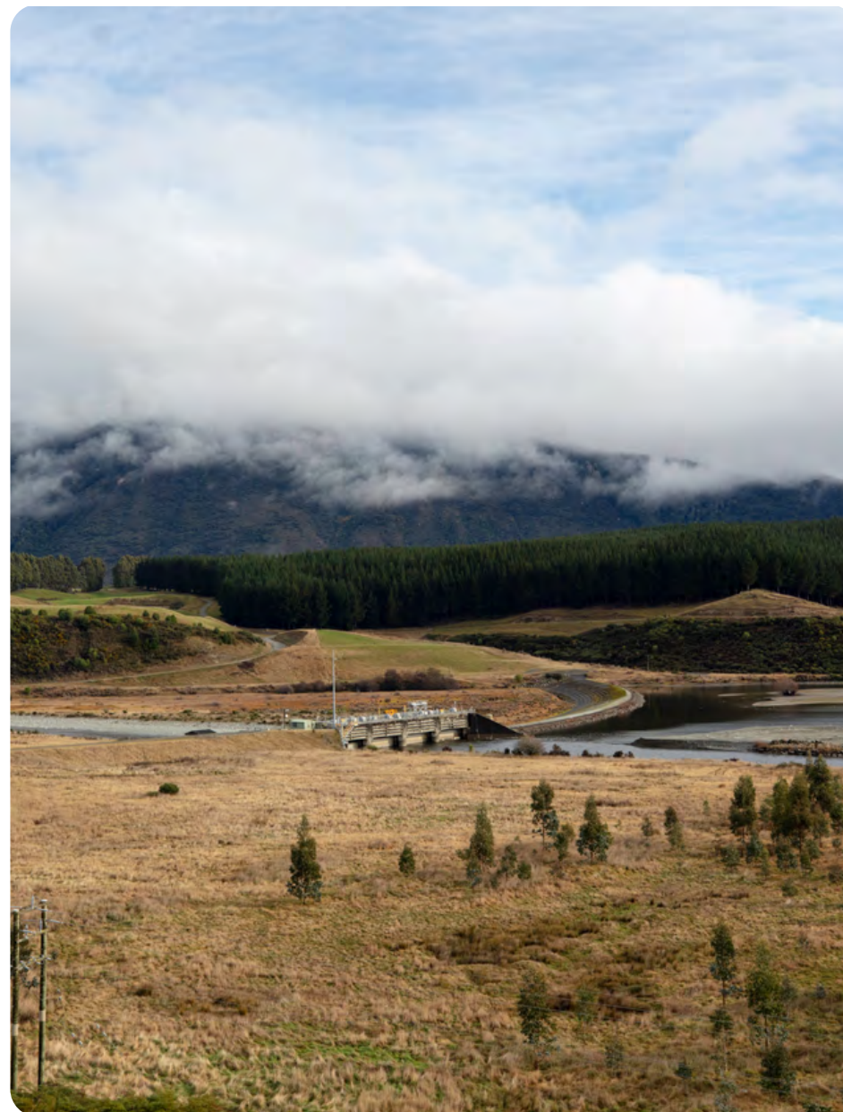
ABOVE: Manapōuri Lake Control Structure, Mararoa Weir.
