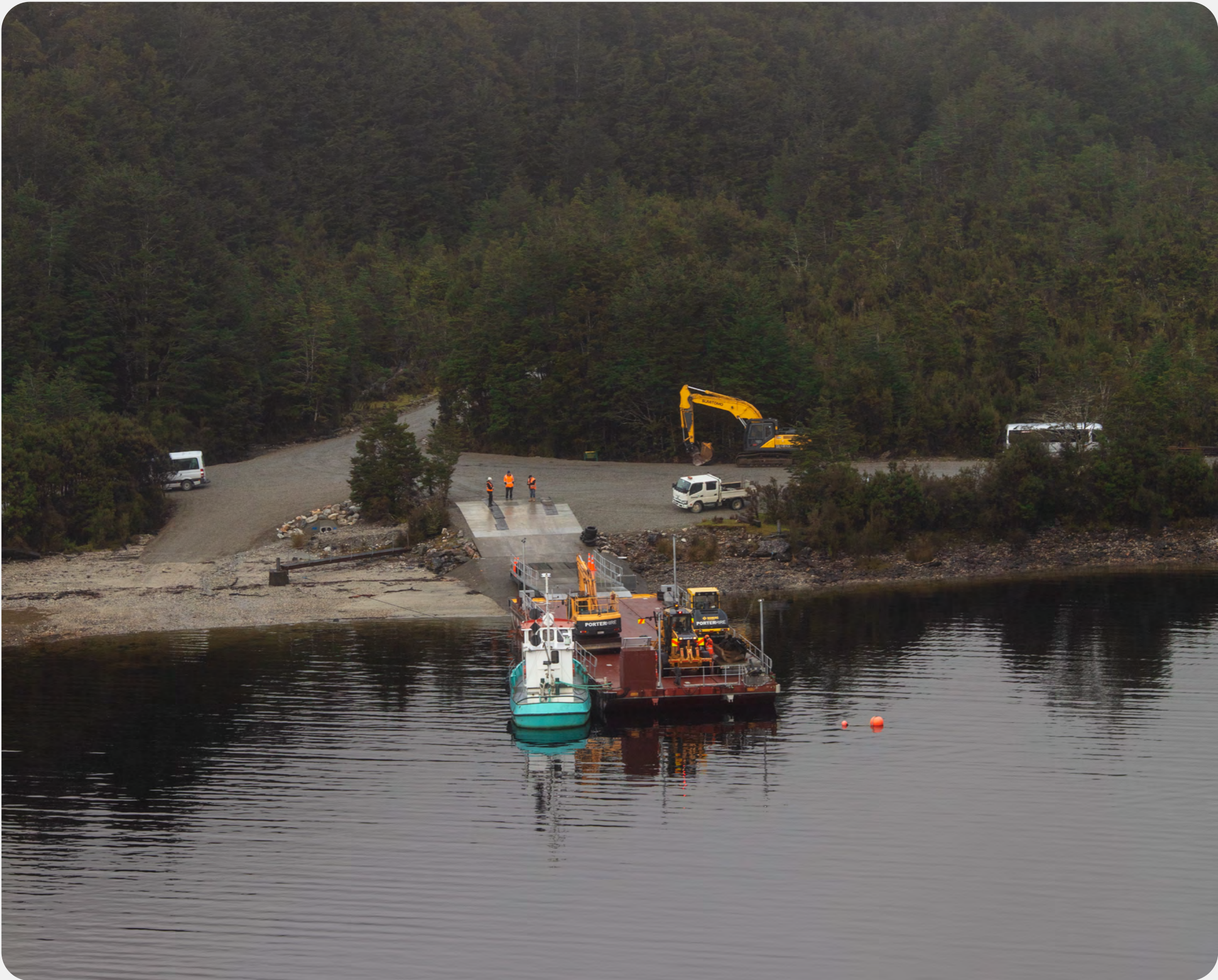
ABOVE: Loading the barge at West Arm, Lake Manapōuri.
