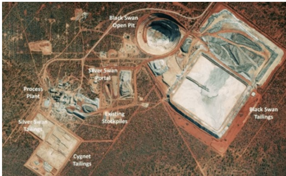
Figure 25 - Black Swan Processing Facility and Associated Infrastructure
