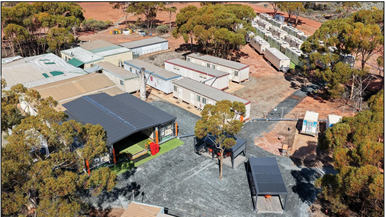
Figure 5 – BSPH expanded Wet & Dry Mess facilities installed on site
