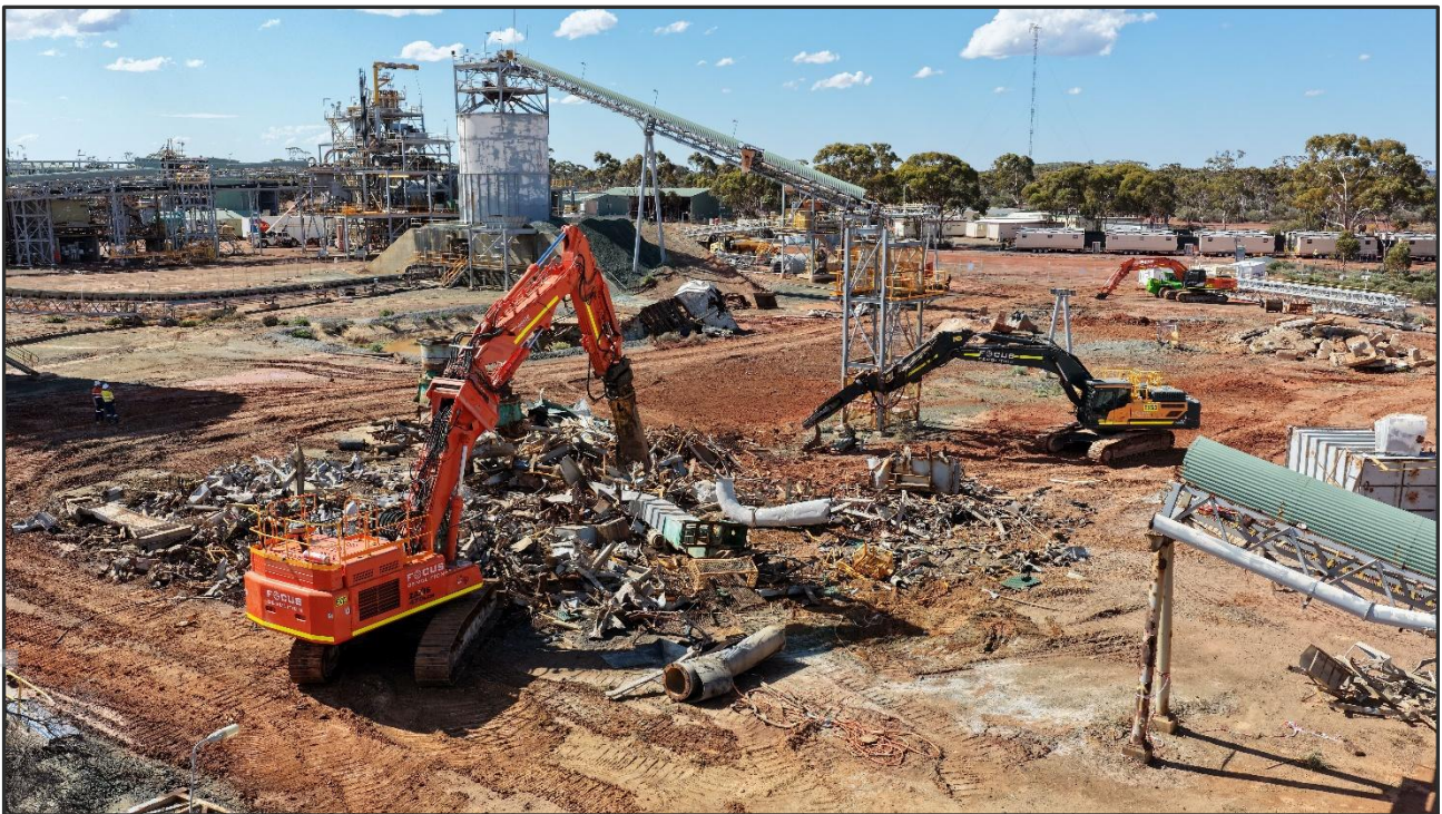
Figure 1 – Demolition of redundant conveyors and structures
