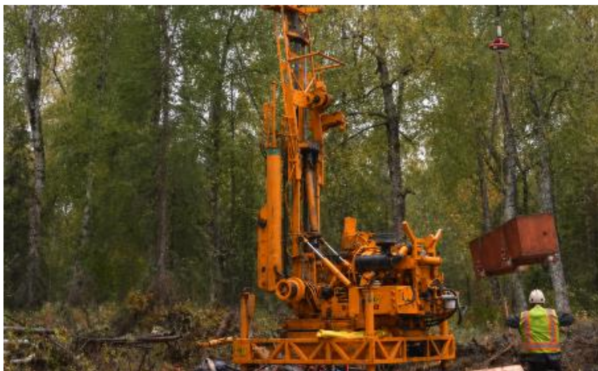
Figure 2. Geotechnical drilling on the West Susitna Access Road route. Source ADOT&PF
