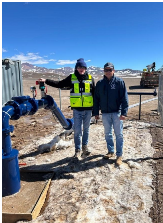
Hydrogeology consultant John McCartney and Chilean Notary inspecting the completed water infrastructure
