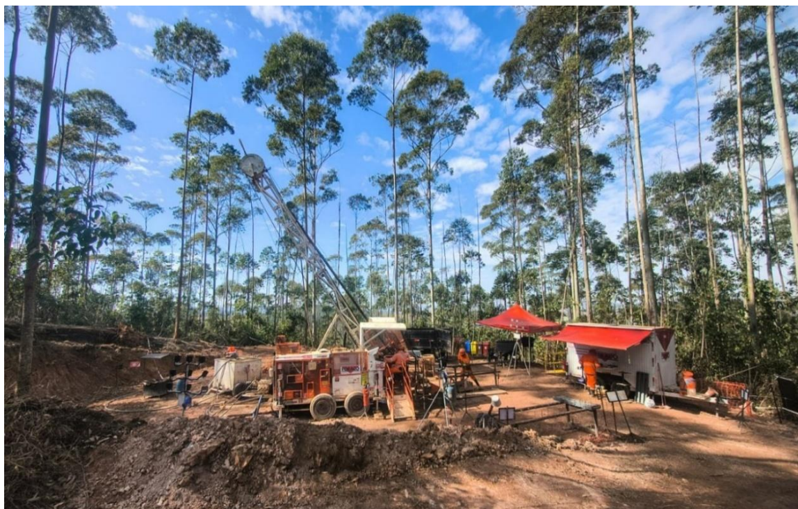
Figure 1. Drill rig on site at the Morro do Ferro project
