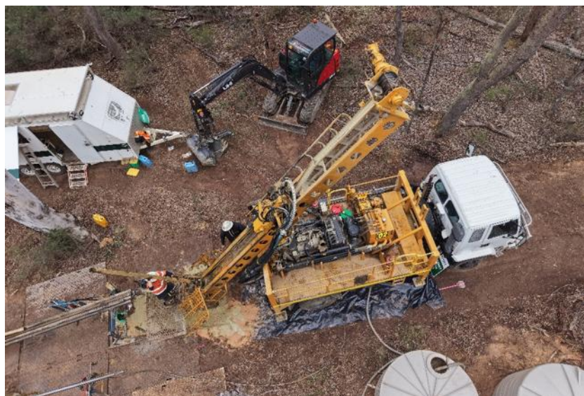
Figure 1. Local contractor Chief Drilling diamond drill rig positioned on the first drill site.
