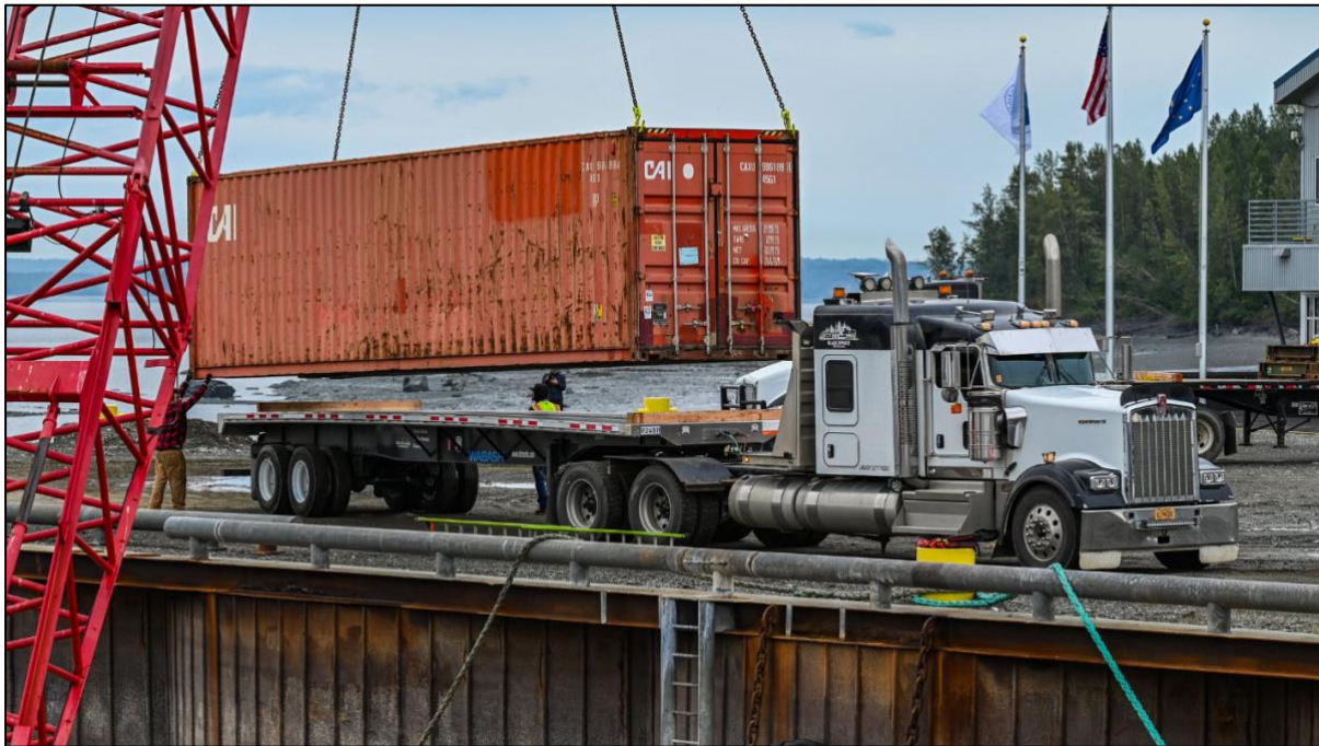
Figure 3. 40ft shipping containers loaded onto trucks for the short haul to the Nova Minerals antimony processing plant site
