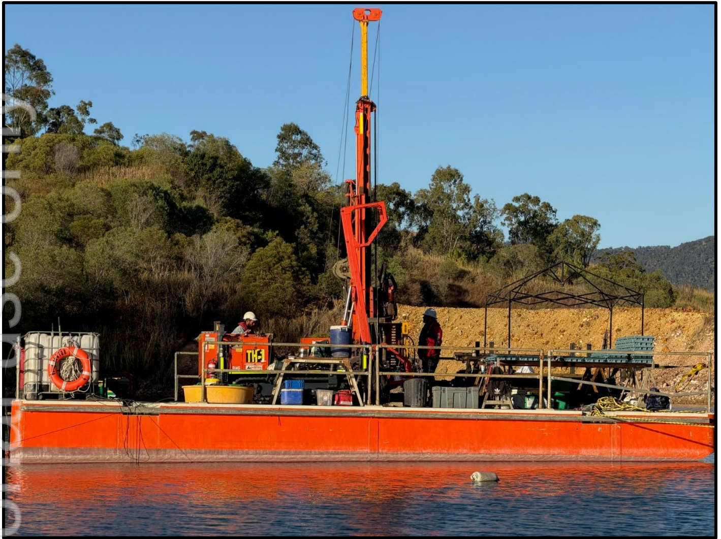
Figure 6 – Rig 19 Barge Drilling.
