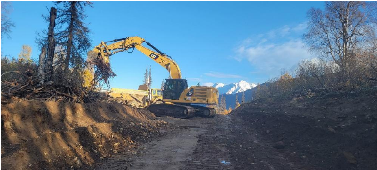
Figure 3. Korbelt-Stibium access road construction works
