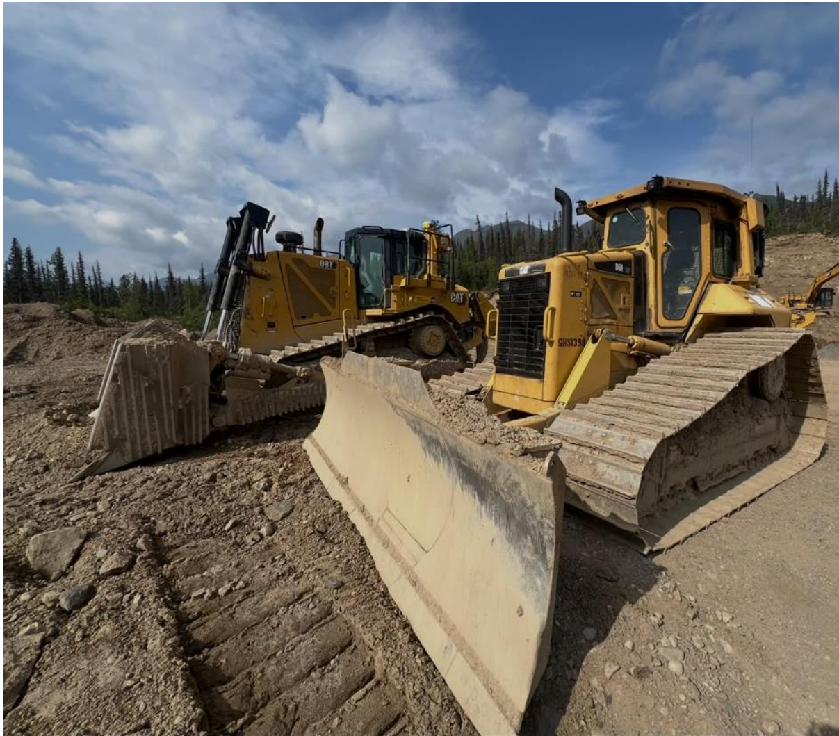
Figure 4. Whiskey Bravo airstrip expansion construction works
