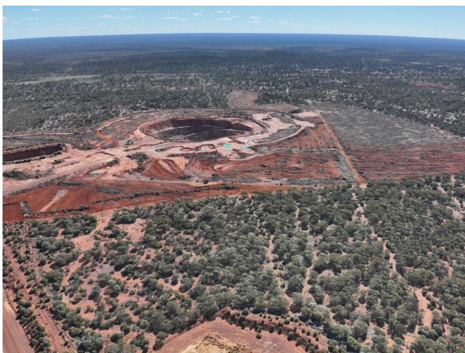
Figure 9 – Lord Byron open pit – existing pit, site establishment works and access roads
