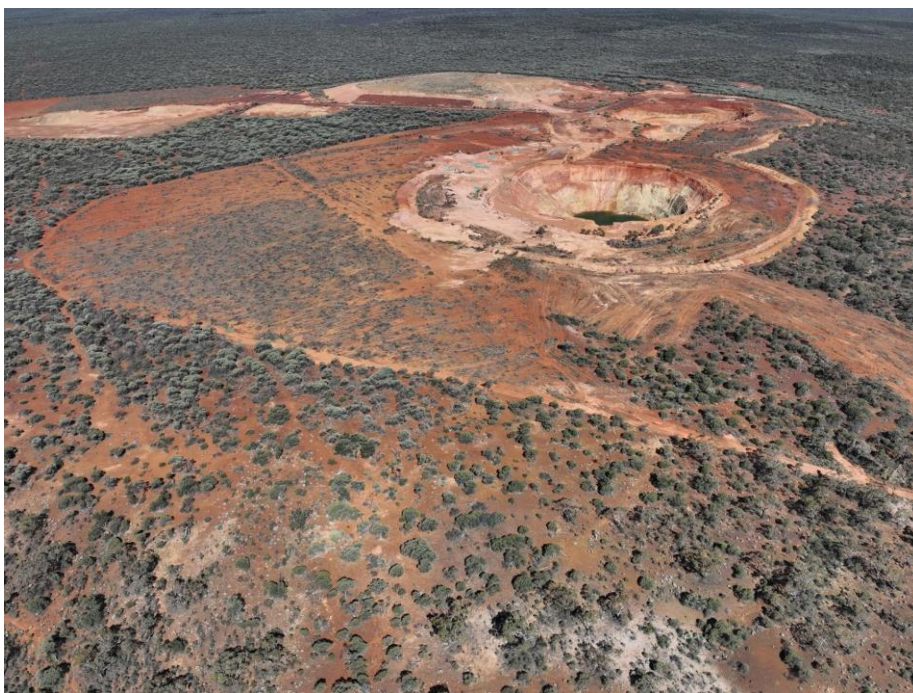
Figure 8 – Lord Byron open pit – site establishment underway
