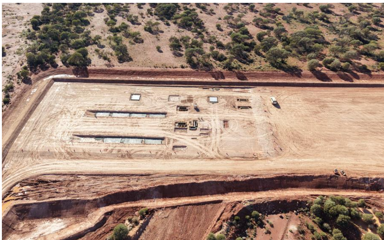
Figure 7 – Power station area – concrete commenced
