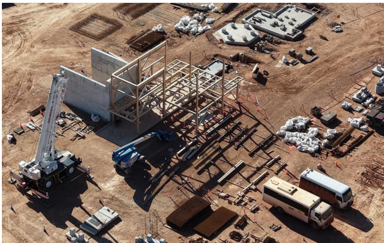
Figure 5 – Surge bin area – structural steel erection commenced
