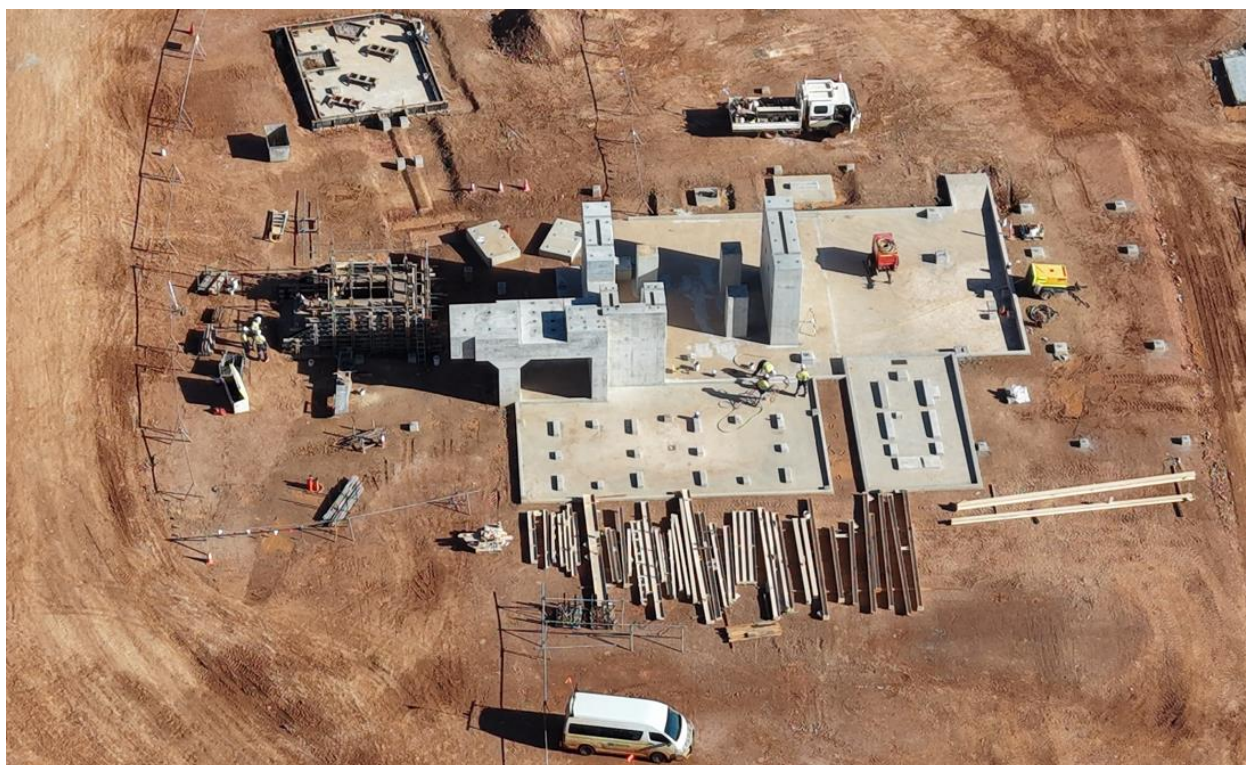
Figure 3 – Grinding and Classification area – structural steel delivered to site and laid out alongside completed concrete ahead of erection
