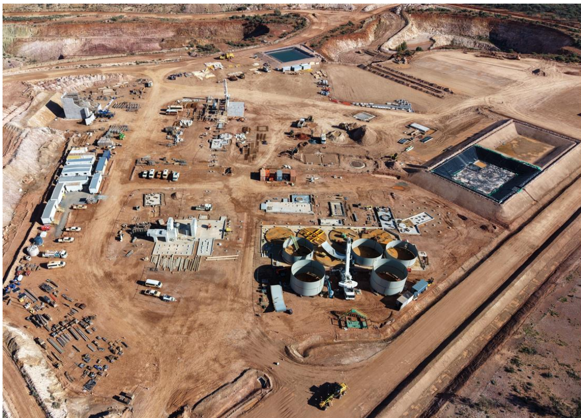
Figure 1 – Process Plant site construction progressing
