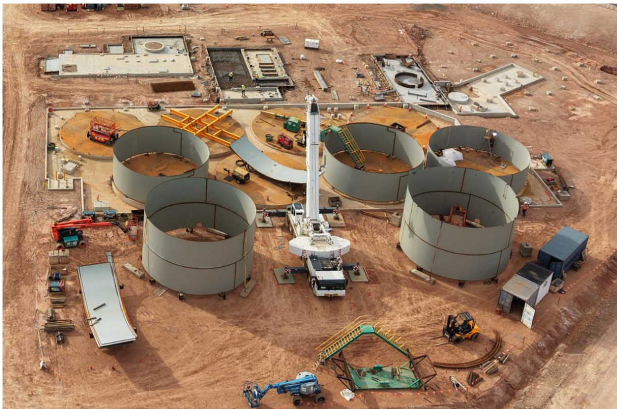
Figure 4 – CIL circuit – tank construction underway
