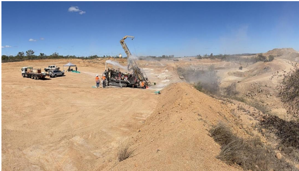
Figure 11: RC drilling underway at Blackjack North Pit
