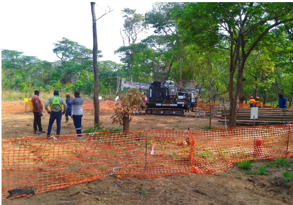
Figure 8. Leos Drilling Rig setting up on first diamond exploration drill hole at Chipimpa
