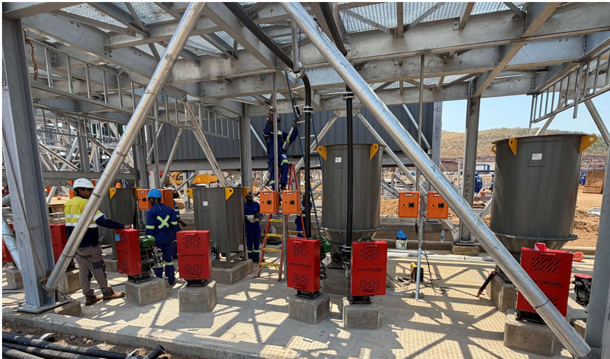
Picture 8. Construction works progressing across the Kangankunde process plant ahead of staged commissioning and first production.
