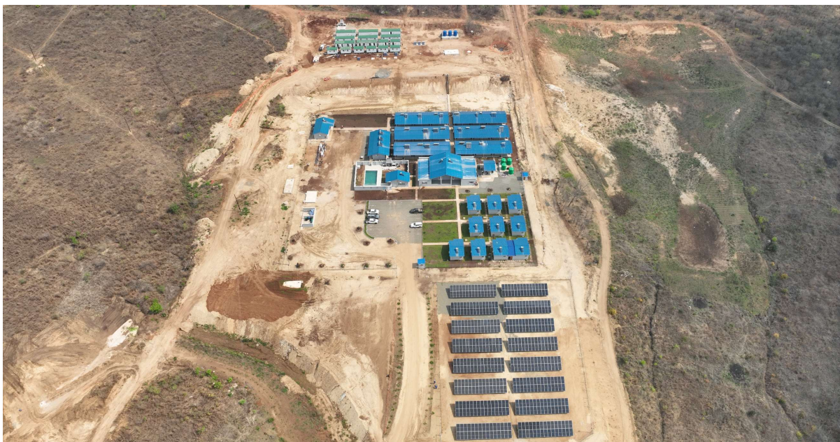
Picture 6. Completed Tipume Accommodation Camp, with expansion works under way to support Stage 1 operations and future Stage 2 development
