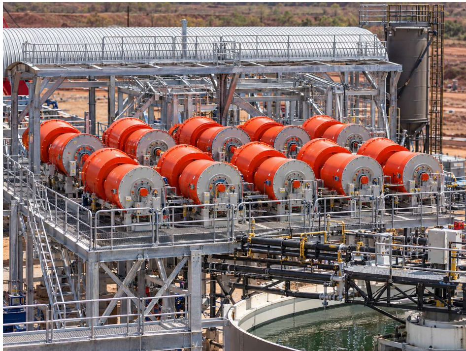
Picture 1. Some of the installation works completed across the Kangankunde process plant's separation circuits ahead of staged commissioning.
