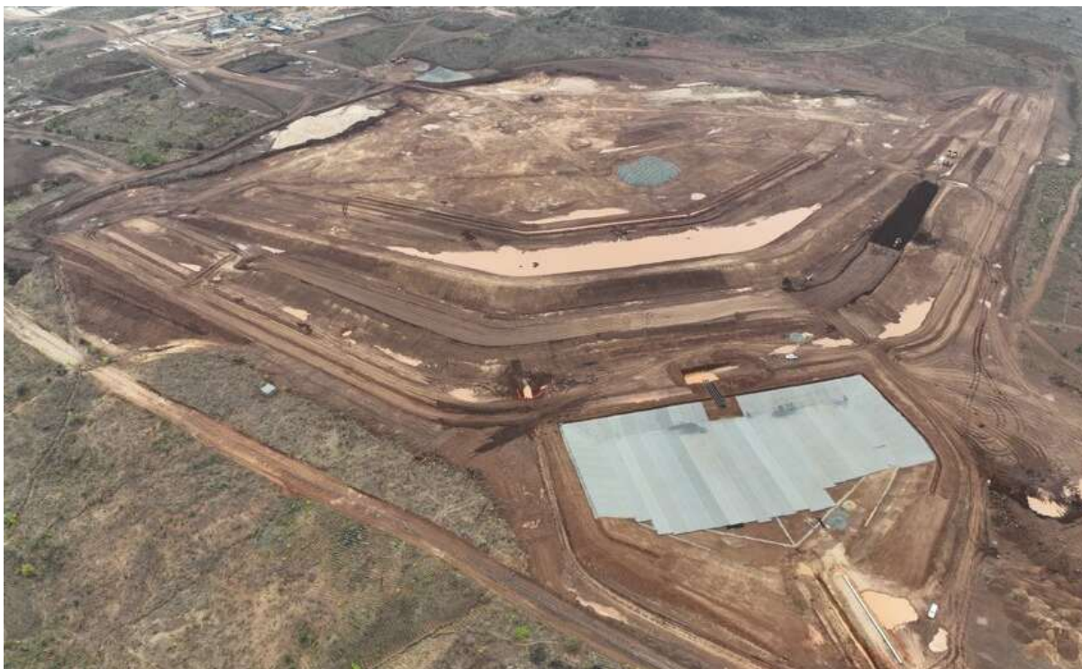
Picture 5. The Kangankunde TSF, with geotextile placement and drainage outfall pipe installation completed
