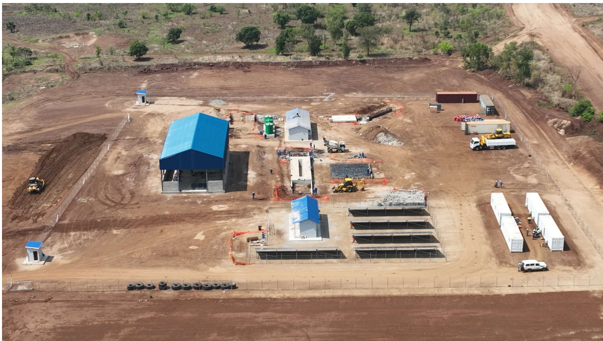
Picture 7. Fuel farm construction progressing alongside the substantially completed HME workshop at Kangankunde
