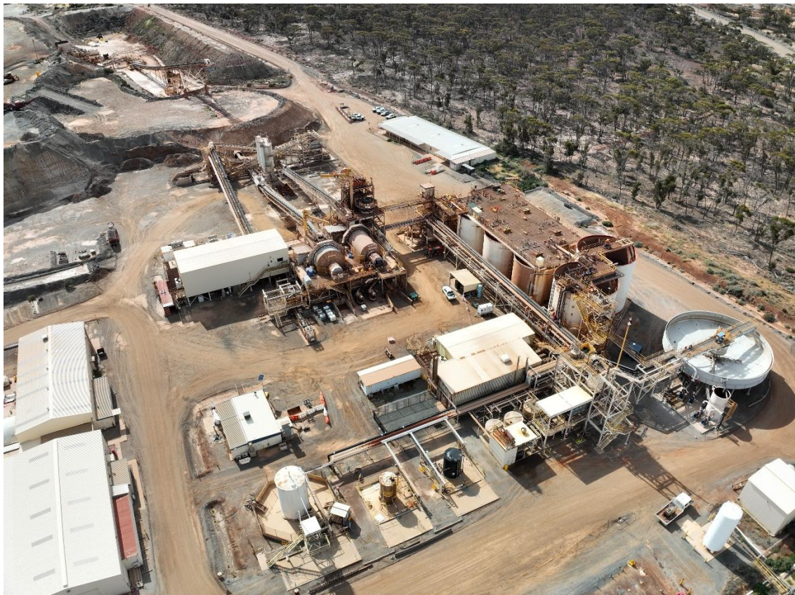
Figure 2: Edna May Processing Facility
