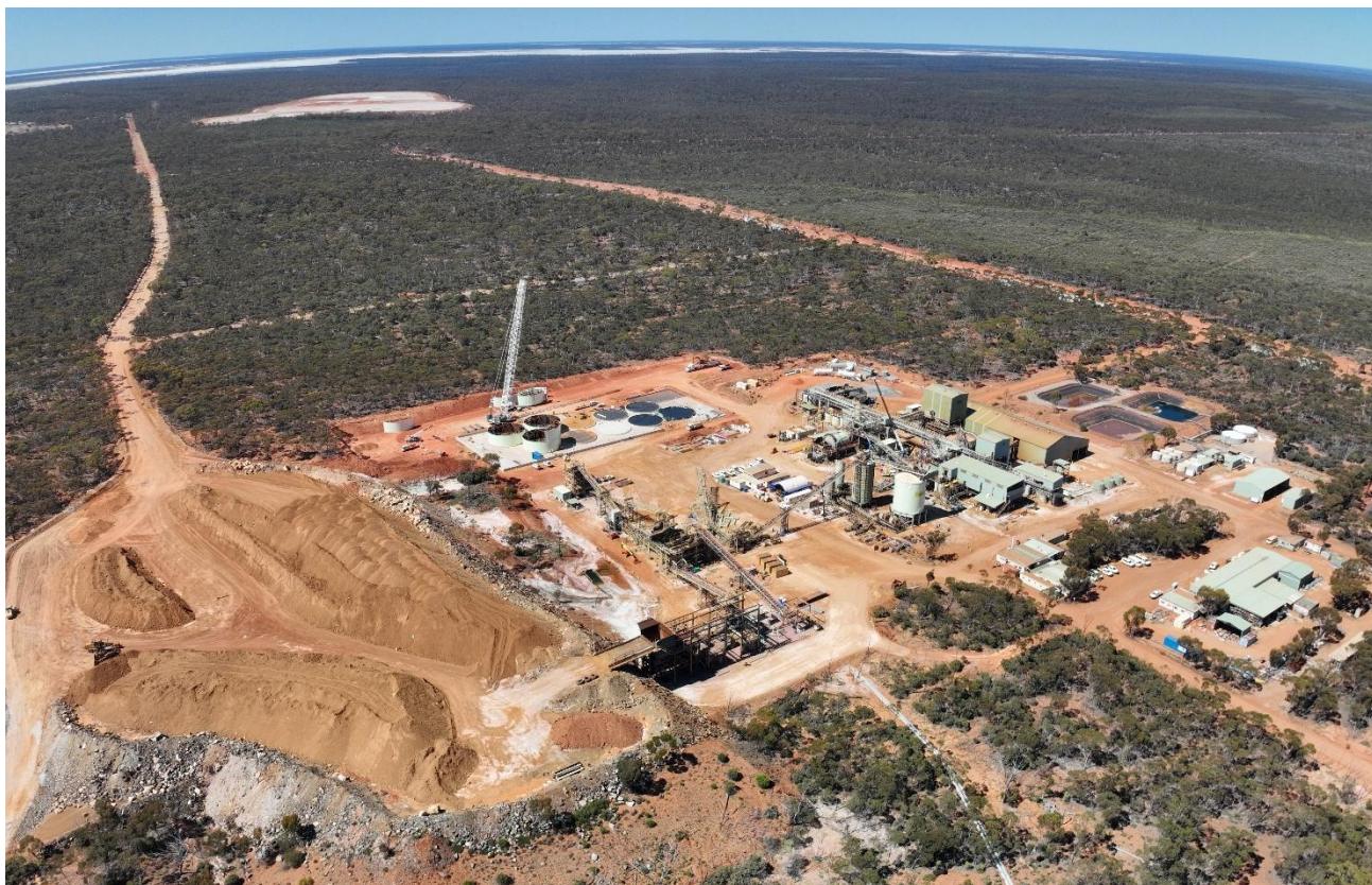
Figure 7: Lake Johnston Processing Facility (~180,000t Lake Johnston ROM Stockpile – left foreground)
