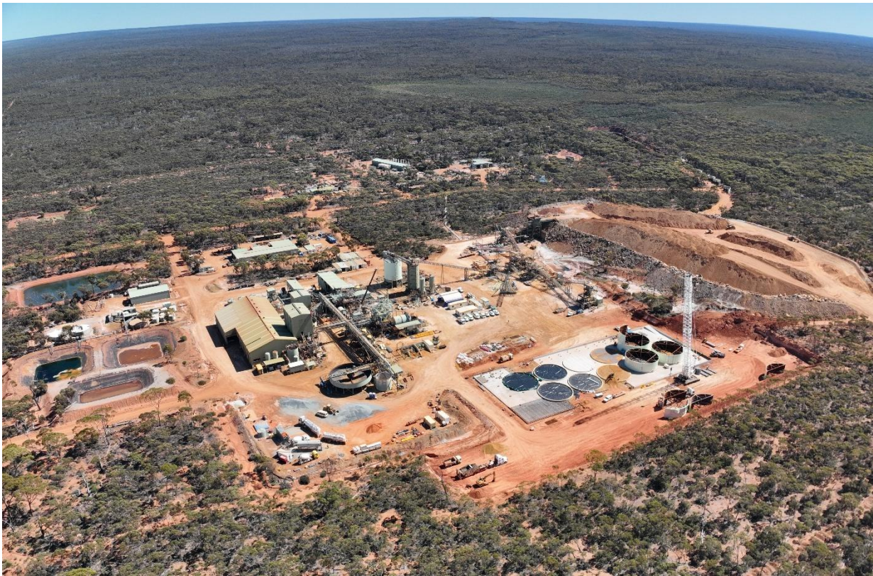
Figure 3: Lake Johnston Processing Facility
