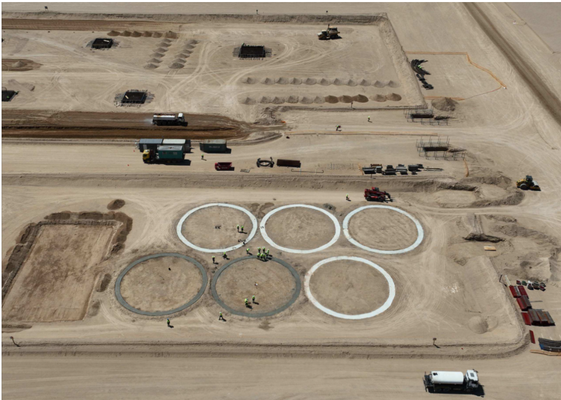
Figure 3: Leach tank ring beam preparations (October 2026).
