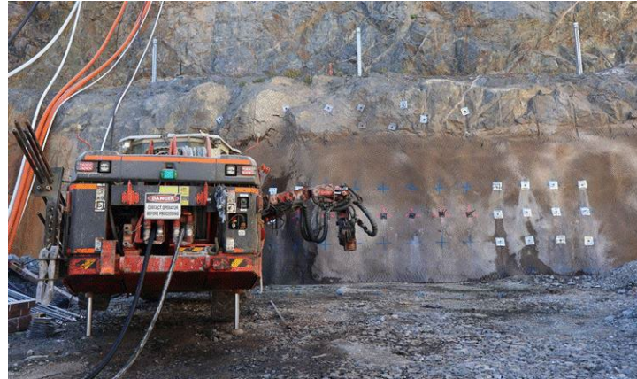
Progress in Kathleen's Corner Underground
