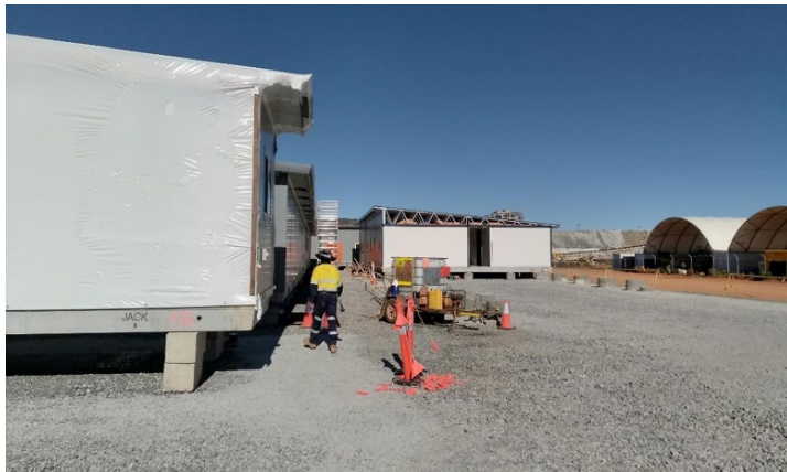
Mine Services Area taking shape
