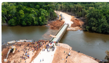
Kido access road, June 2026.
