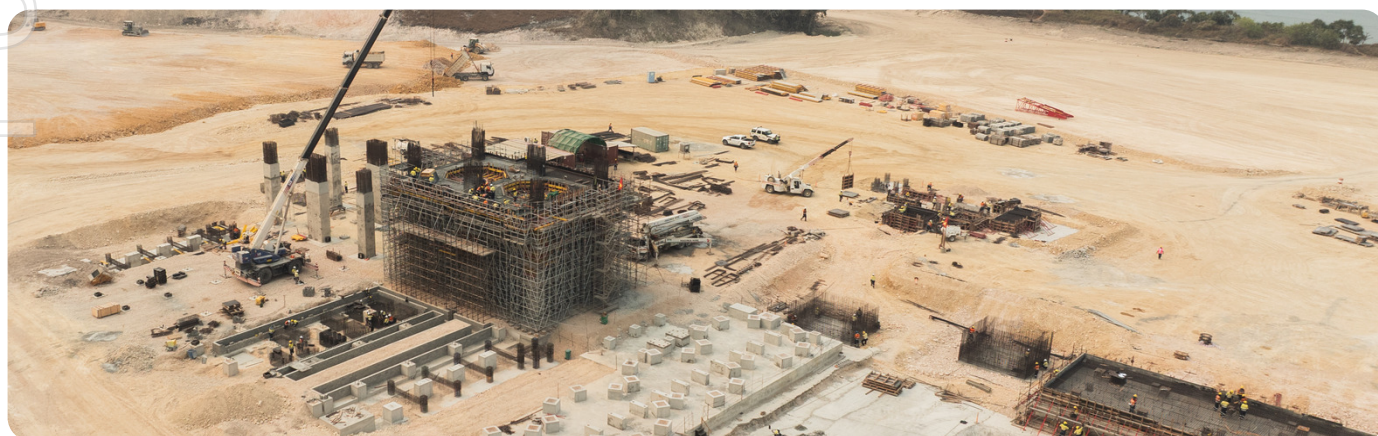
Image: Kiln 1 and Kiln 2 support structures (left), with blower room and lime silo foundations (right)
