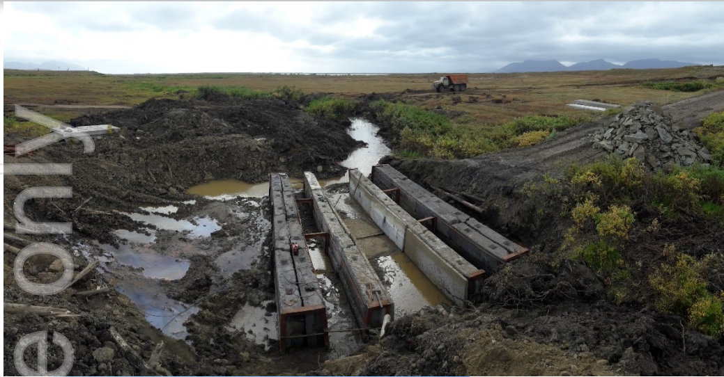
Construction of culverts and stream crossings
