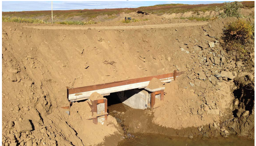
Construction of culverts and stream crossings
