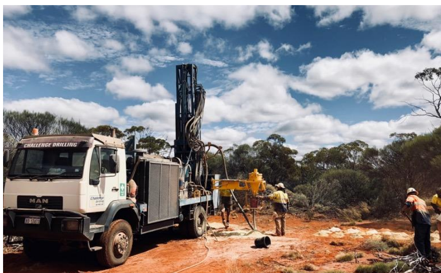
Figure 3 – Aircore drilling at the T8 prospect
